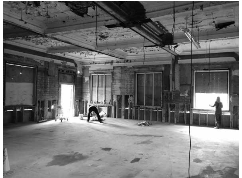
The second floor took a while longer.
